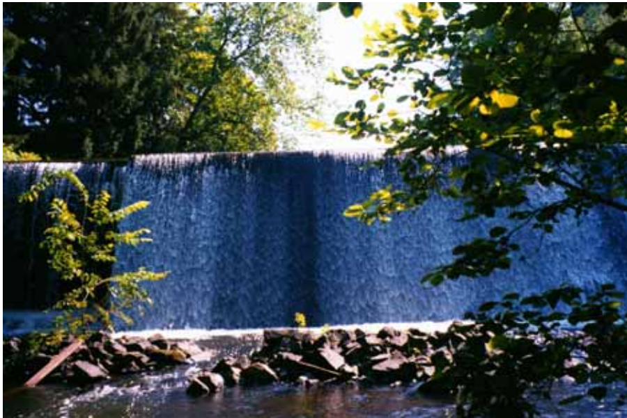
Six dams were noted in the seven Tankerhoosen River segments (5+ miles) surveyed, pointing to the need to address obstruction of fish passage in the River.
