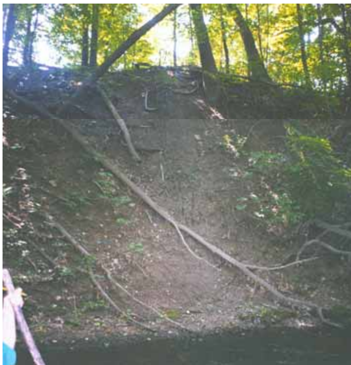
This eroded streambank was found in Segment 7, upstream of Route 83. The bank was 30-35 feet high, and nearly vertical. Surveyors did not note any human (or other) activity that might be causing the slope to erode.
