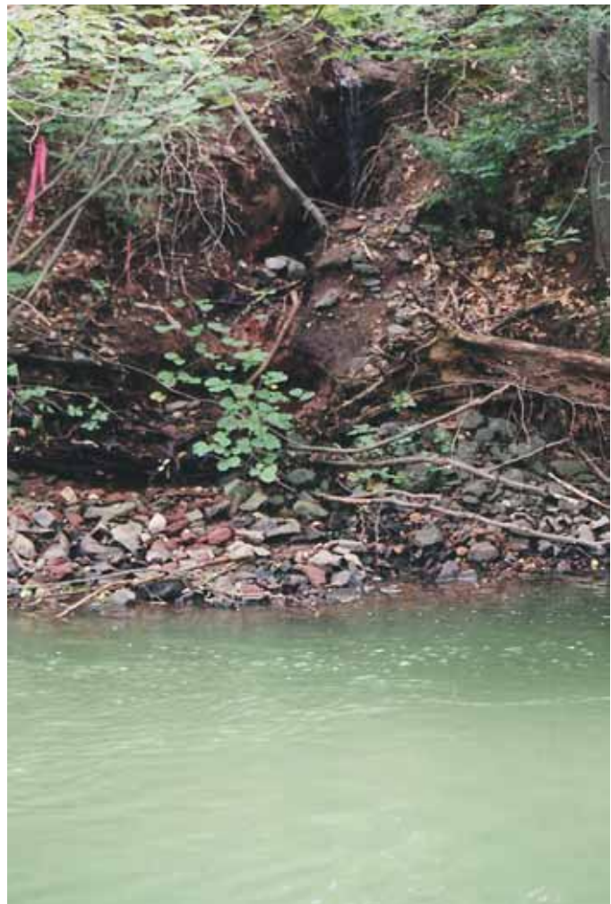
Along a Hockanum River segment in Manchester, this erosional gully was formed on the stream bank as a result of runoff from a storm drain. The greenish tinge to the water is due to an algae bloom that occurred during the summer drought.
